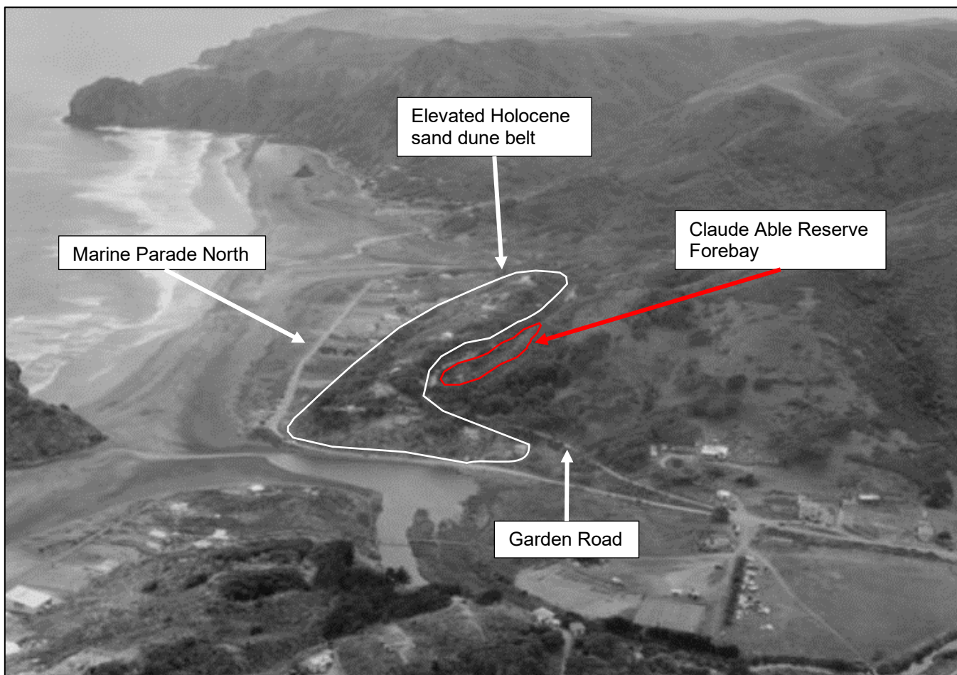
Figure 2.2: Oblique aerial image taken in 1955 showing the elevated, Holocene sand dune belt and the approximate location of the Claude Able Reserve Forebay (source: White Aviation Ltd).
