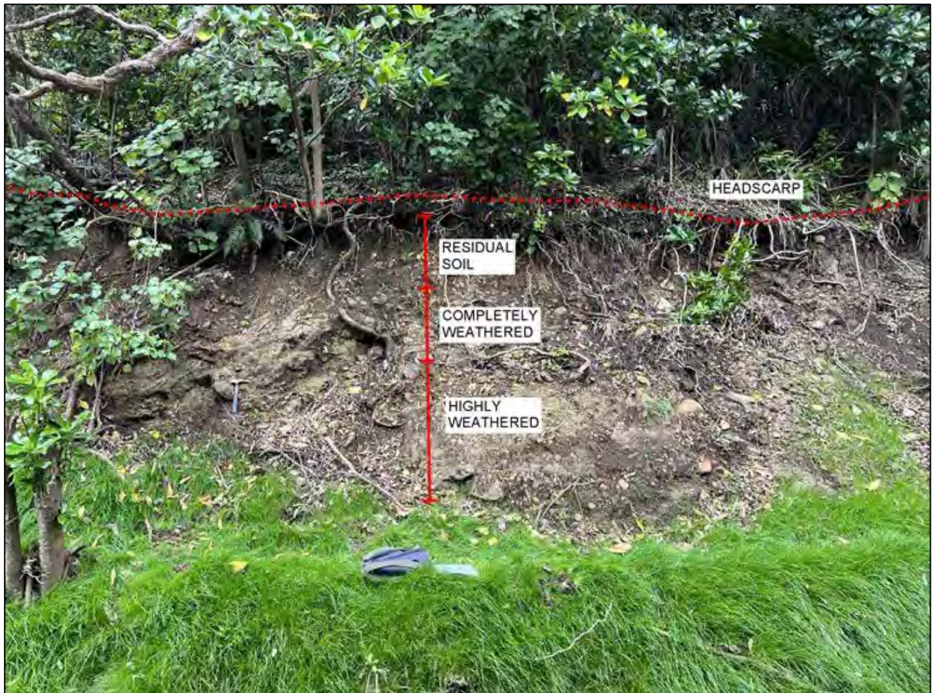
Figure 2.9 Example of the typical weathering profile in Piha Formation.
