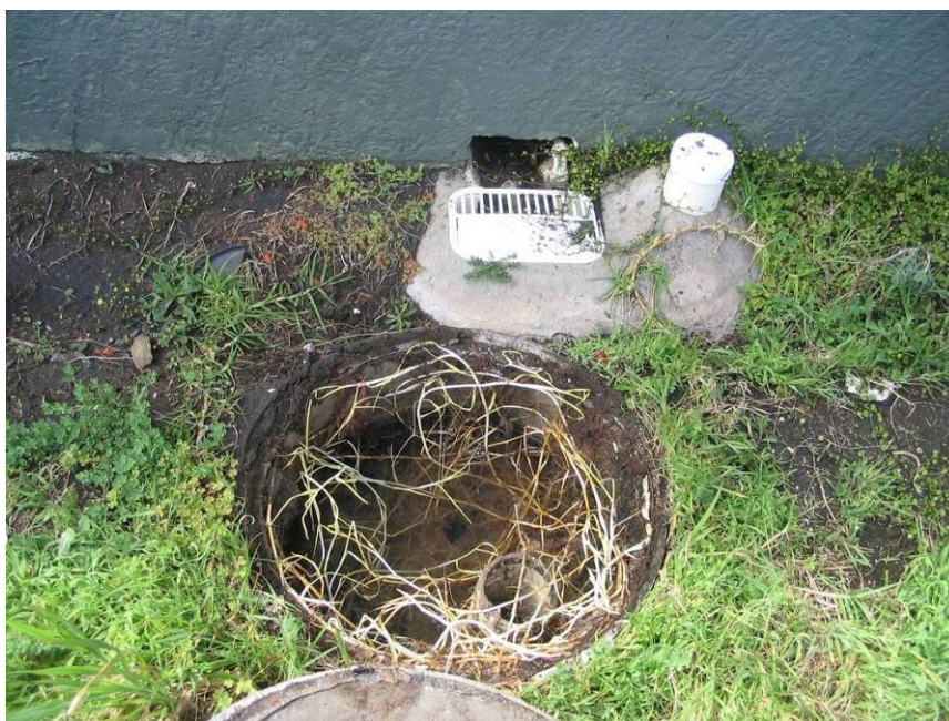
Root intrusion clogging a septic tank system, Piha area
