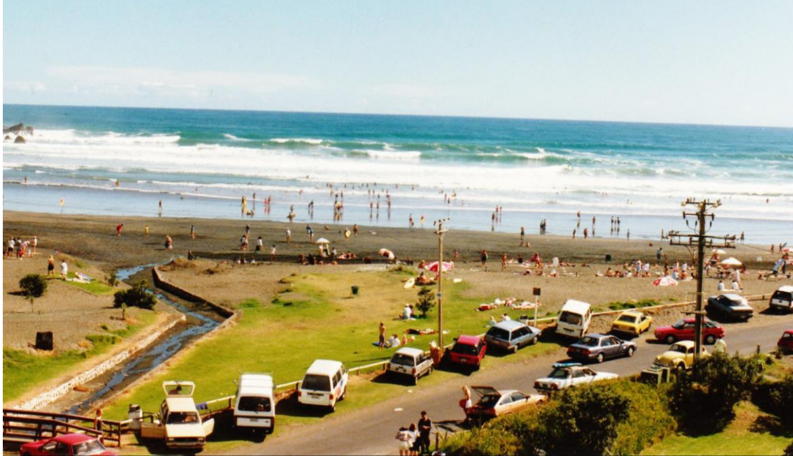
Figure 5: Moana Stream in 31 March 1991 subsequent to training (concrete lining) of stream (1984-5) which eliminated the earlier flared entrance to create a larger grassed amenity area. This photo was taken prior to construction of the along dunes along seaward margin and it can be clearly seen that beach views from the reserve were then quite expansive (Photo supplied by Mr Barry Davis).
