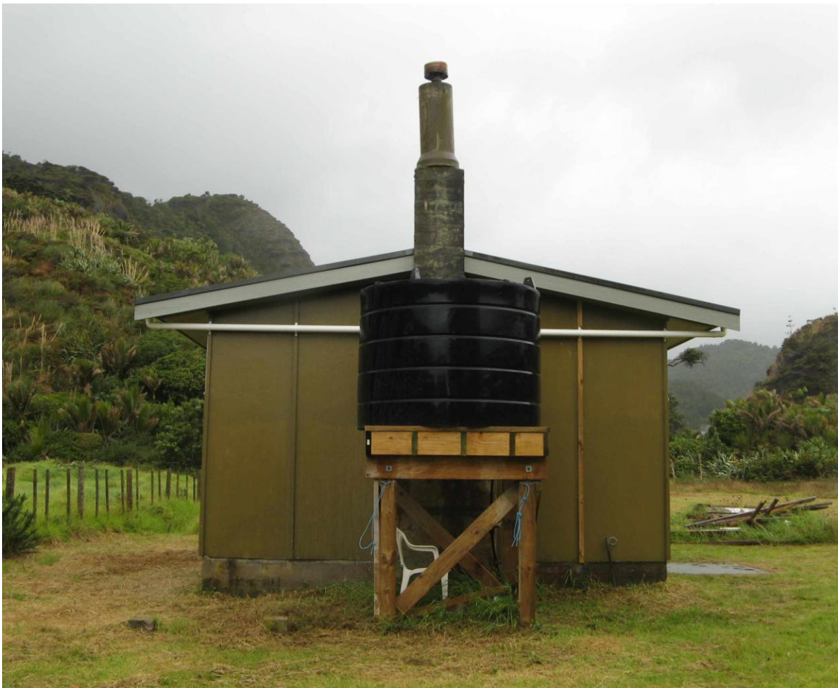
Figure 6: West elevation showing pre-cast concrete chimney, with its extension, a concrete drain pipe, and the recently repaired tank stand.
