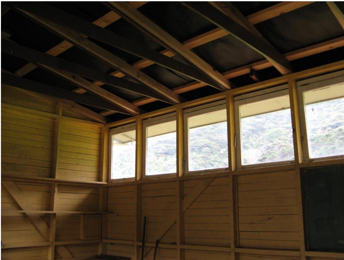
Figure 8: Detail of interior walls and clerestory windows.
