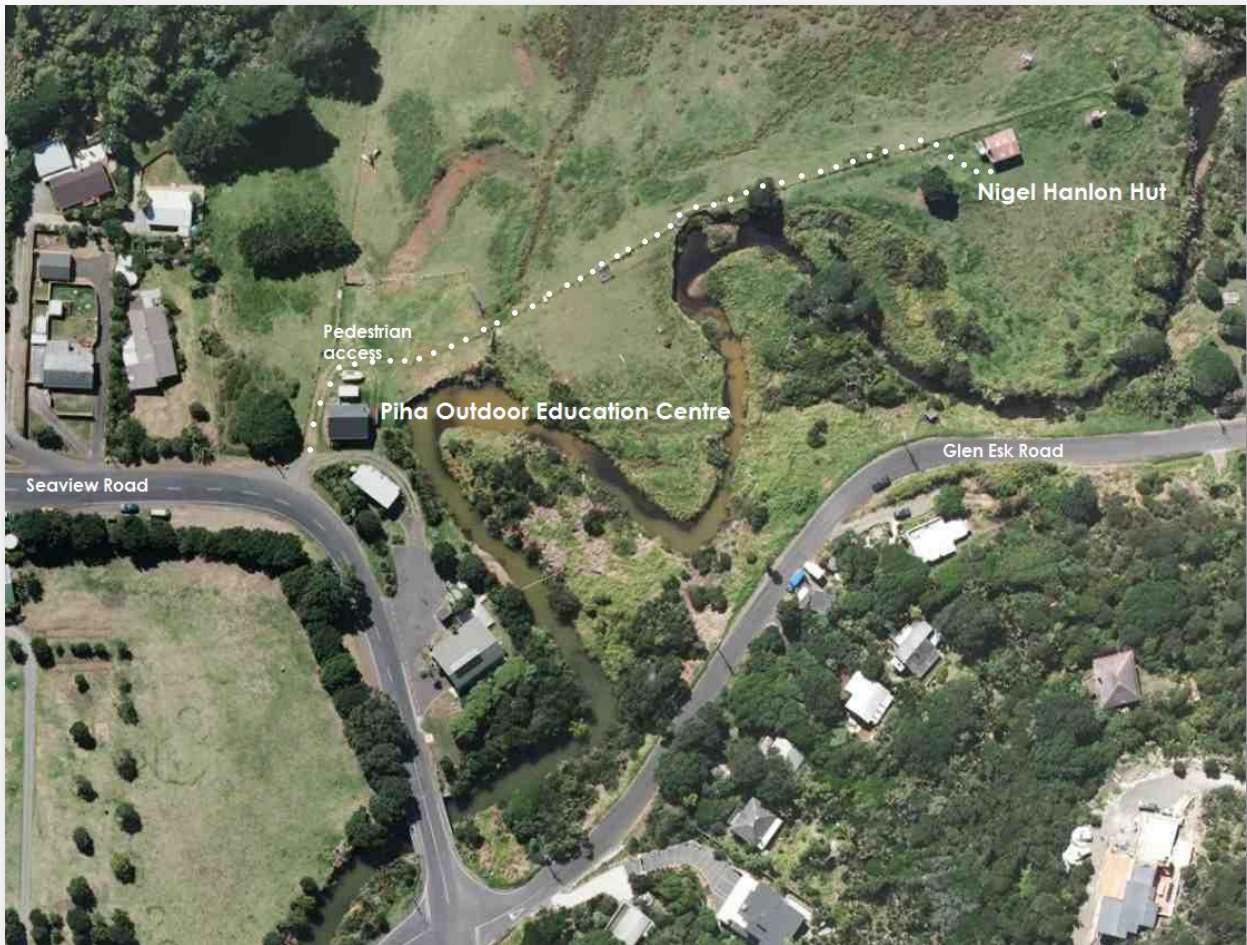
Figure 1: Location of Nigel Hanlon Memorial Hut showing access through the former Piha School (Piha Outdoor Education Centre) land. Source: ALGGI Website
