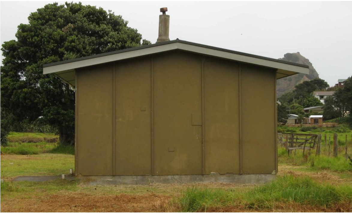
Figure 5: East elevation showing past repairs to the fibrolite cladding.
