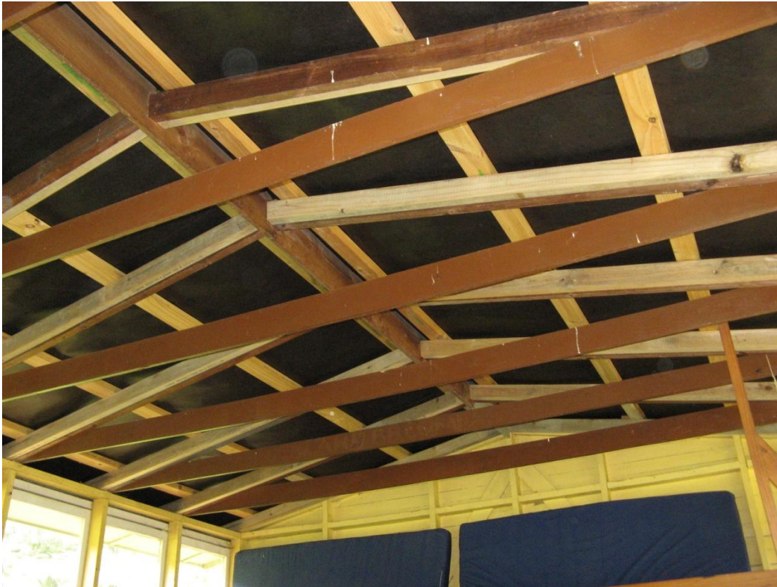
Figure 7: Roof framing showing replacement purlins and new rafters inserted alongside original work.
