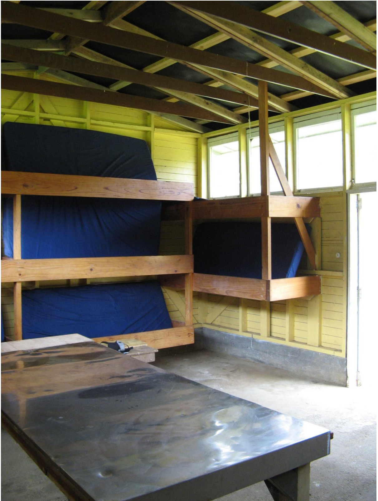
Figure 11: Tiered bunks on the east wall.
