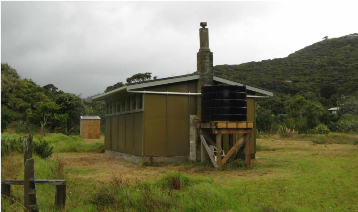
Figure 2: Nigel Hanlon hut (north and west elevations) and its associated re-built double long-drop privy.
